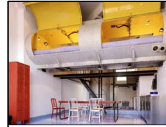
CARVING OUT AN OIL TANK 4 HATCHBACK DOORS CUT FROM BOTH SIDES OF THE TANK ARE OPENED BY HYDRAULIC PISTONS TO OFFER SUNLIGHT AND VENTILATION
