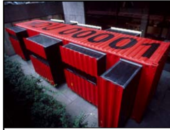
EXTRUDING SPACE WHEN IN USE, ALL SUB-VOLUMES ARE PUSHED OUT, LEAVING THE INTERIOR OF THE CONTAINER COMPLETELY UNOBSTRUCTED.
