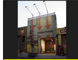
CYNTHIA BROAN GALLERY - NEW YORK THE FACADE IS A THIN LAYER OF PRINTABLE VINYL MESH THAT IS DRAPED OVER THE OLD BRICK WALL CREATING AN ADDITIONAL EVER-CHANGING ART
