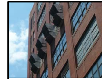
ADAPTING EXISTING TECHNOLOGIES THE STAINLESS STEEL EXTRUSIONS WITH LARGE GLAZED FRONTS ARE MADE WITH THE TECHNOLOGY OF AIR DUCTS PROTRUDING OUT OF
