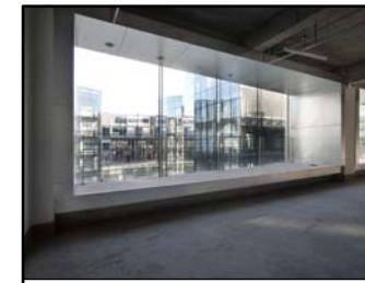
CONNECTING INDOOR AND OUTDOOR THE STEEL EXTRUSIONS FUNCTION AS ENTRANCE, DISPLAY AND BAY WINDOWS AND EXTEND THE INTERIOR SPACE/PROGRAM ONTO THE PIAZZA
