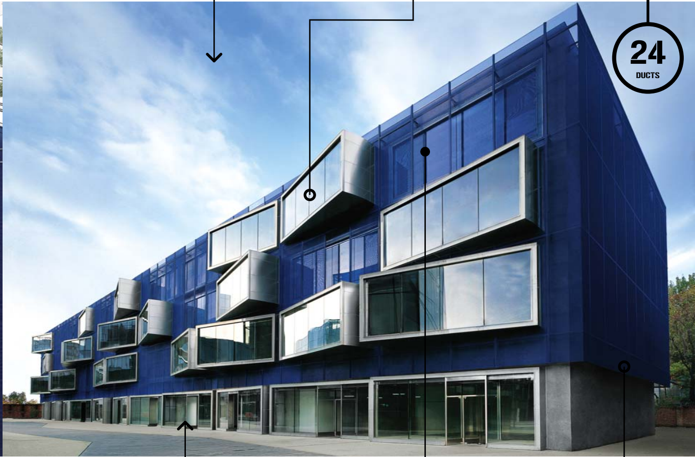
ACTIVATING WITH LIGHT + MOVEMENT LARGE EXTRUSIONS PIERCE THE MESH AND BEND WITH VARYING ANGLES. AT NIGHT, THE EXTRUSIONS BECOME LIGHT BOXES WITH LED FRAMES
