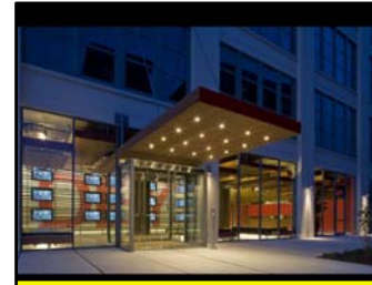
CANCO LOBBY - JERSEY CITY, NJ THE VAST LOBBY OF THE CANCO LOFTS BECOMES A DYNAMIC PUBLIC SPACE AND A PULSATING PRESENCE WITHIN THE REVITALIZATION OF JERSEY
