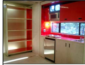
PULLING OUT STORAGE ROLLING BOOKSHELVES AND CLOSETS OPEN INTO THE CENTRAL VOLUME OF THE CONTAINER.
