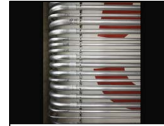
BENDING ELECTRIC CONDUIT A SCREEN MADE OUT OF BENT ELECTRIC CONDUIT SUPPORTS AND FEEDS THE TECHNOLOGICAL INFRASTRUCTURE AND DEFINES THE SPACE
