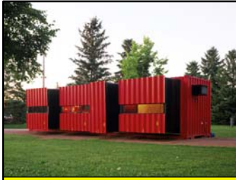
MOBILE DWELLING UNIT - WHITNEY MUSEUM CUTS IN THE METAL WALLS OF THE CONTAINER GENERATE SUB-VOLUMES, EACH ENCAPSULATING ONE LIVE, WORK OR STORAGE FUNCTION
